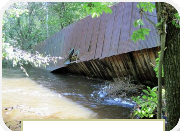
Turkey Jim Bridge in the water.
