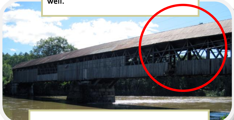
The water was very high to get through the side of Blair Bridge.
