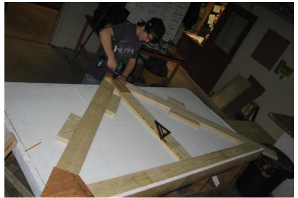
Trusses being fabricated..... re-calculating the pitch of the roof
